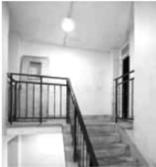
photo of stairwell with LED fitting
