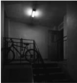
photo of stairwell with fluorescent fitting
