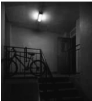
photo of stairwell with fluorescent fitting
