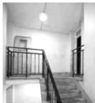
photo of stairwell with LED fitting
